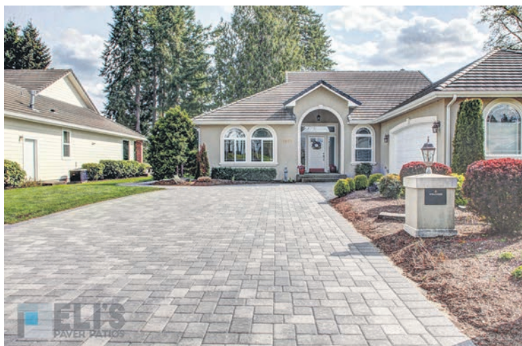
A finished project done by Eli's Paver Patios.
